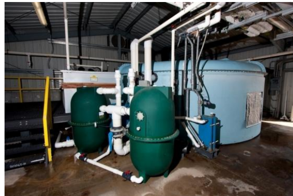
Figure 3. Newly designed and constructed recirculating maturation system for WSB.
